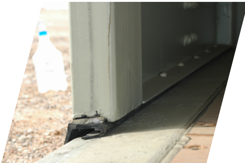
Figure 5. Note rubber gasket in door jam between steel door and steel floor. Superworms would tightly appress themselves against this rubber seal and avoid exposure to the fogging application. Many survivors were recovered from this area.
